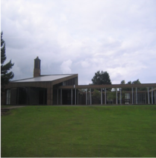
Crematorium general view
